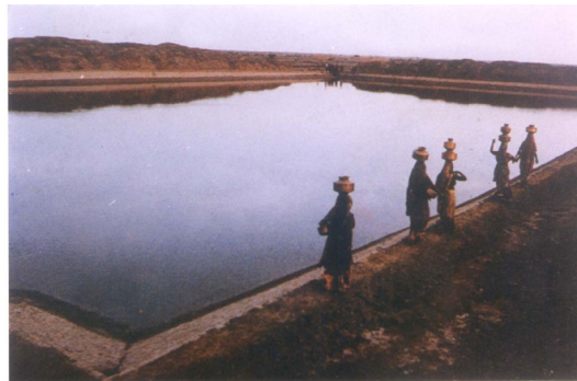
A pond lined with Low Density Polyethylene (LDPE) to collect and store water
