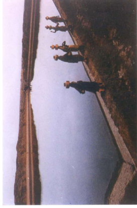
A pond lined with Low Density Polyethylene (LDPE) to collect and store water
